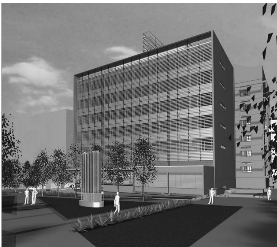
Just completed is a new state of the art biology research building. This is an exciting time for research in Biology and the new facility will greatly enhance our ability to carry out leading edge research.
